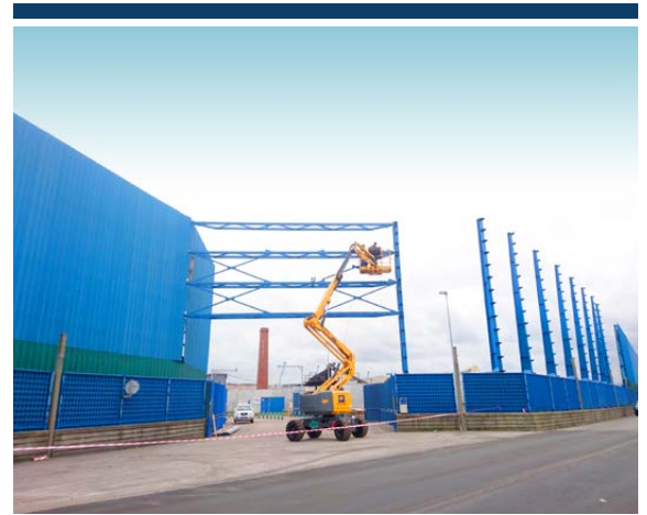
Modular, movable, porous, anti-pollution shield Door1 (left bank). August 2018 / 600 l.m Leylandii anti-pollution tree shield. December 2017
