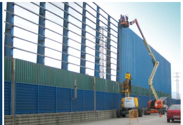
Pantalla opaca fija encierre perimetral del Puerto. Mayo 2015 / Fixed opaque shield at the perimeter enclosure of the Port. May 2015
