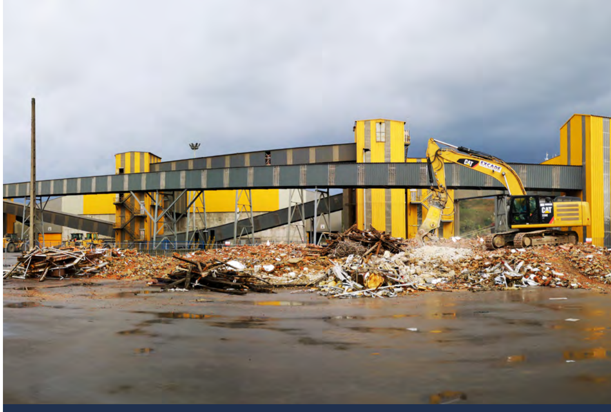
Demolición del Antiguo edificio de Estiba (SEAVED) Demolition of the Former Stowage building (SEAVED)
