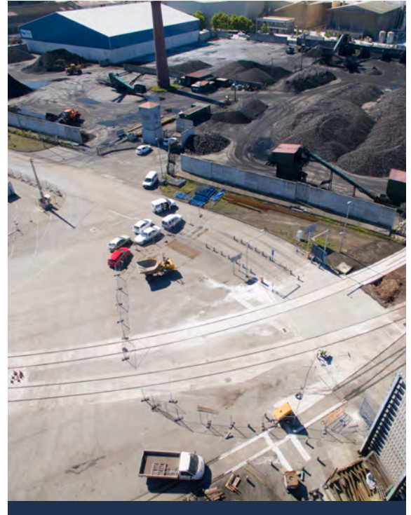
Vista aérea de un tramo del nuevo anillo ferroviario terminado Overhead view of a segment of the new completed ring rail line
